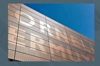
Contrast can be achieved on an expanded metal mesh by simply rotating the mesh upside down.
